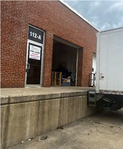
View Dock & Entrance
