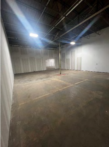
Interior View Side Room
