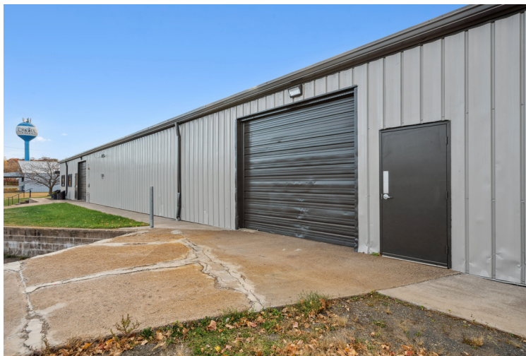
Drive-in Door with Platform Dock on North Side
