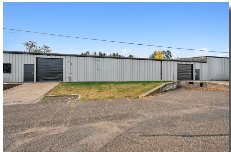
2 Drive-in Doors on East Side
