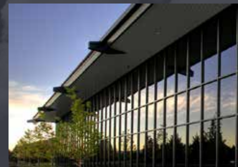
5390 Kietzke Lane, Reno 65,917 SF Class A Office
