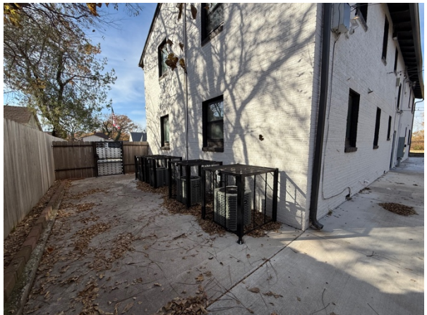
Covered AC Compressor units.
