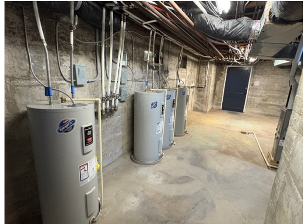
Basement hot water heaters.
