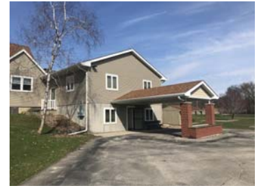
Private Entry of Premises
