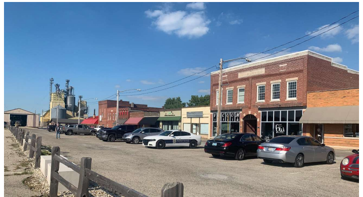
Existing Buildings Downtown Bargsville
