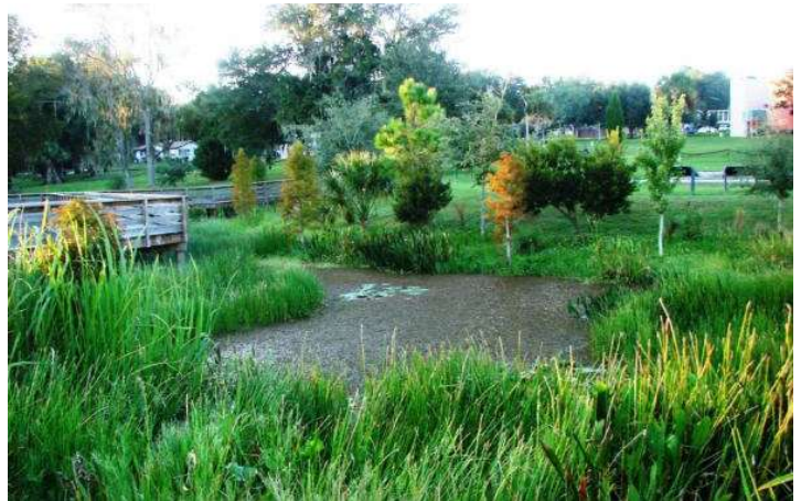
Constructed wetland stormwater facility adjacent to a residential development, Source: Geocaching.com
