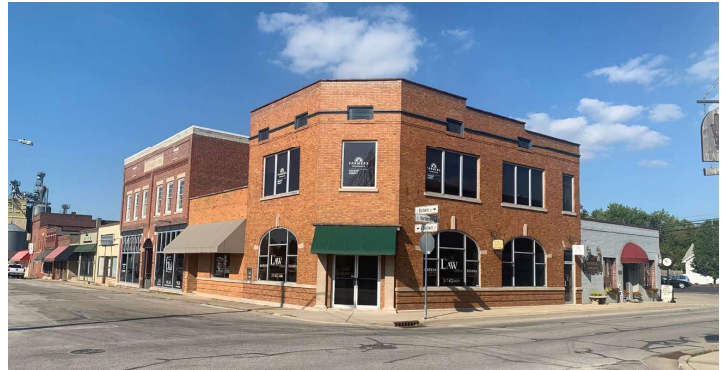
Existing Buildings Downtown Bargsville
