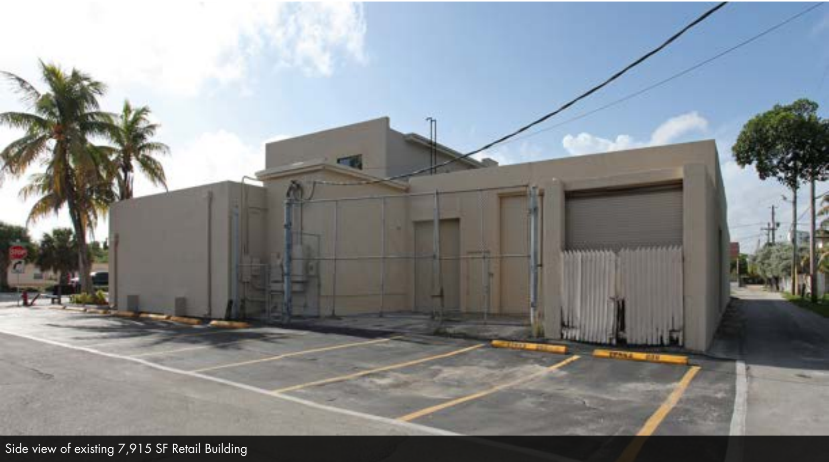
Existing 7,915 SF Retail Building
