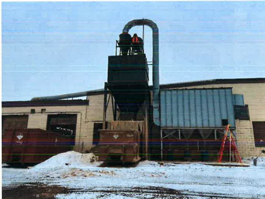
Photo 10 Looking north at the dust collection unit located south of Building A, January 2024.
