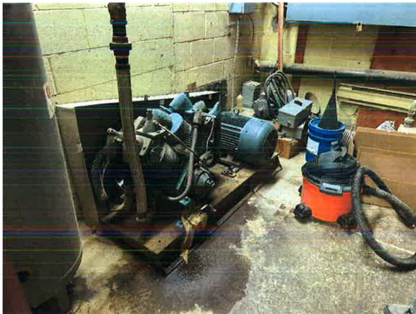
Photo 6 Compressor and adjacent small leak inside Building A, January 2024.
