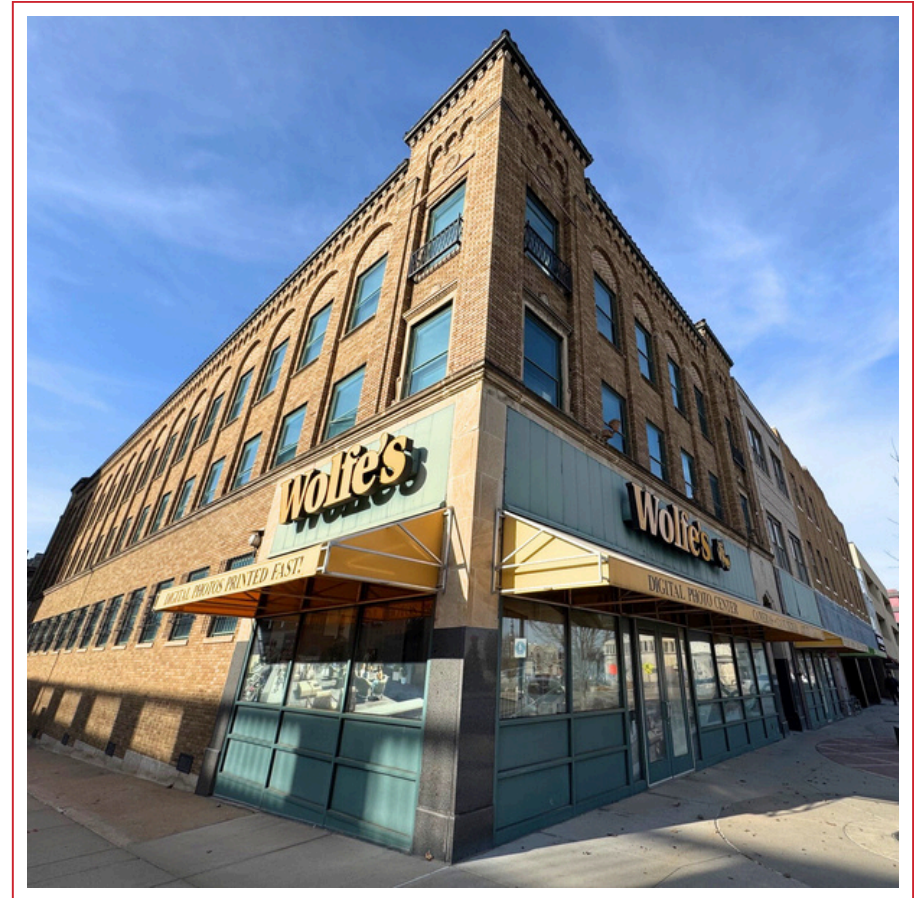
Corner Retail & Garage Parking
