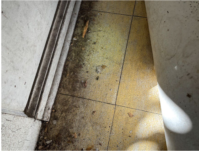
Photo 3: 12"x12" Floor Tile, Tan (ACM) and Associated Mastic (ACM) in 2 nd floor Kitchen under linoleum sheeting
