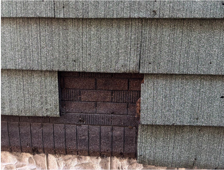
Photo 1: Exterior Brown Shingle Siding (ACM), Exterior of House
