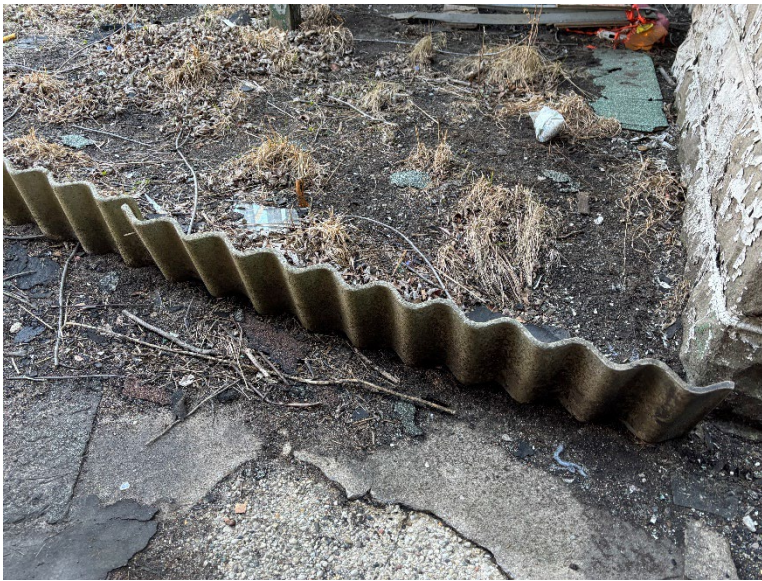
Photo 2: Transite landscape fencing (ACM), Exterior West side of House
