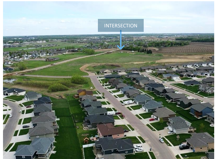
Above 54 th Street facing South East towards Marion and Benson Intersection
