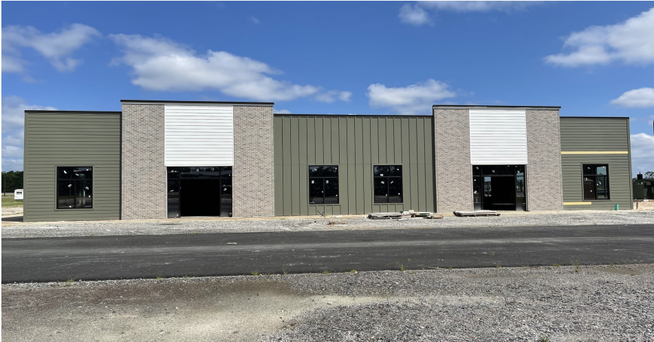
Retail Building Construction Photo - 3rd Quarter Delivery
