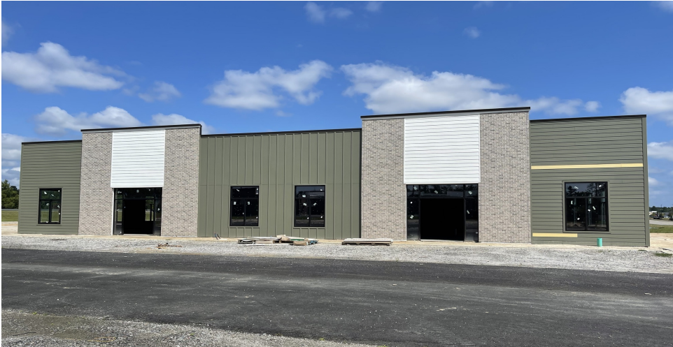
Retail Building Construction Photo - 3rd Quarter Delivery
