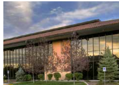
5370 Kietzke Lane, Reno 55,559 SF Class A Office
