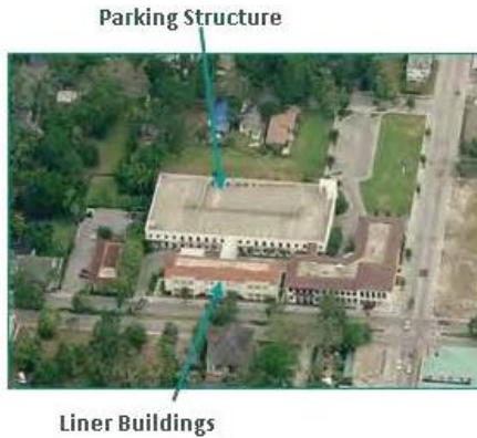
Figure 18. Detached Liner Building
