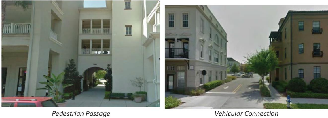
Pedestrian Passage Vehicular Connection Figure Notes: Floors above walkway not required. Photos are illustrative, not regulatory ( Ord. No. 2994 , § XVI, 3-15-2023)
