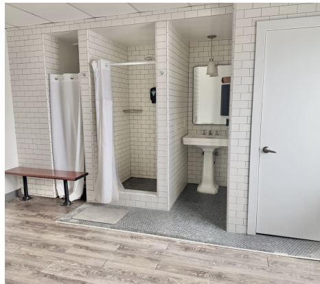
Existing locker / shower facilities
