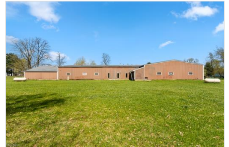
Back of Structure
