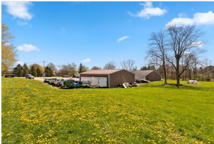
Back of Structure
