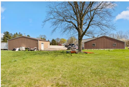
Back of Structure
