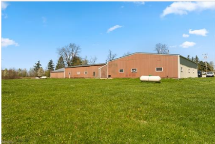
Back of Structure
