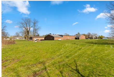
Back of Structure
