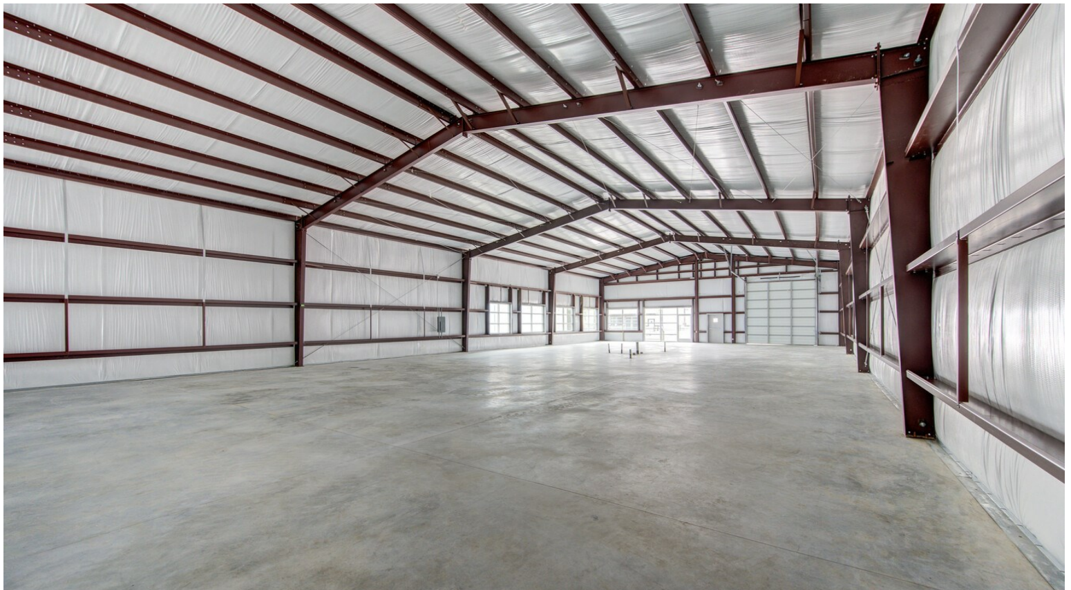
Room for Truck Entry
