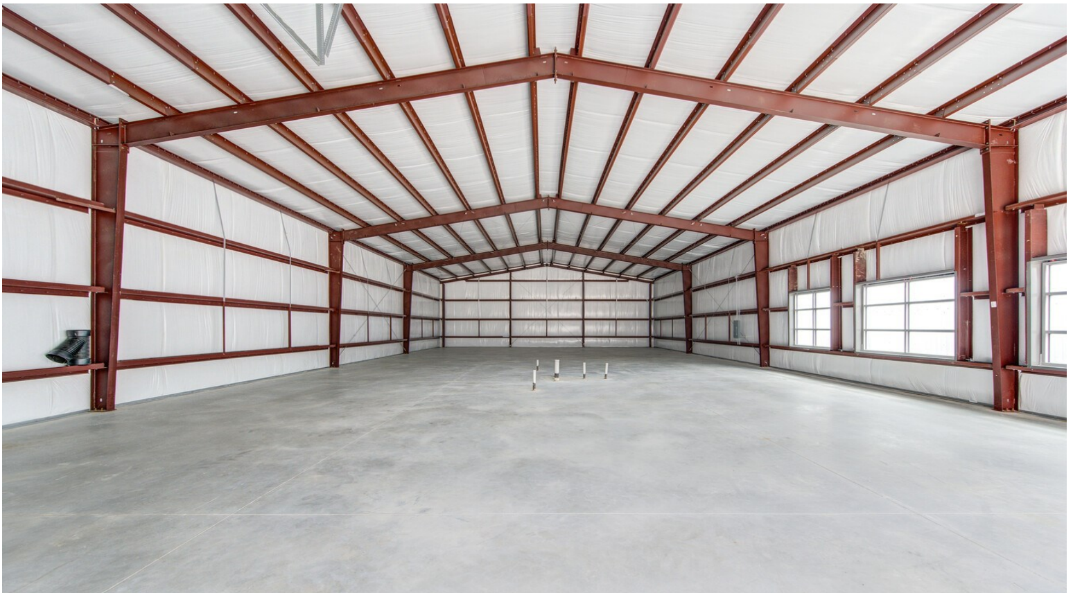
At the Crossroads of Sam Houston Tollway (Beltway 8) and Interstate 69
