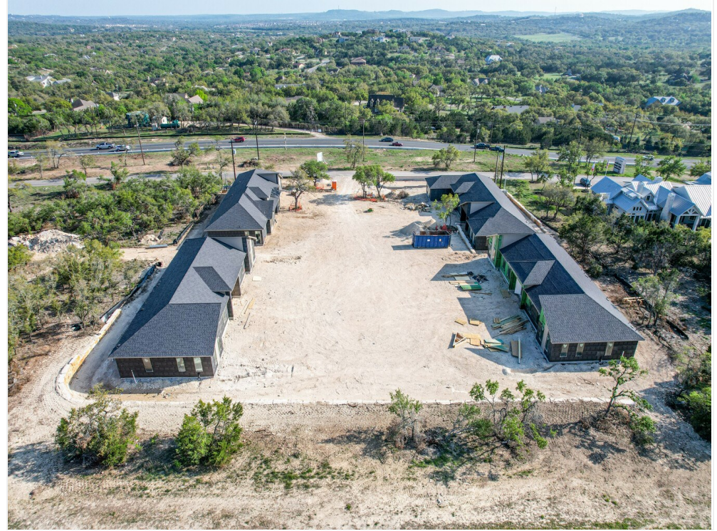
Aerial of Buildings 1, 2, 3 & 4
