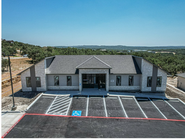
Newly Constructed Building 3
