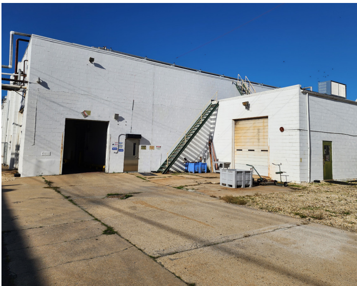
Building 3 (Refrigerated) ± 11,592 sqft 1 Drive-in - 20' Ceiling Height
