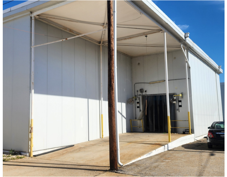
Building 2 (Refrigerated) ± 13,320 sqft 1 Drive-in - 20' Ceiling Height
