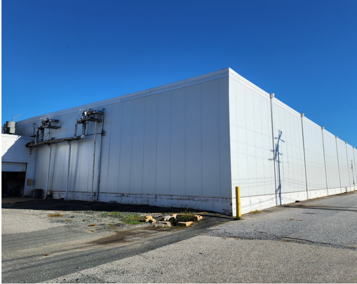
Building 1 (Refrigerated) ± 26,344 sqft 2 Docks - 20' Ceiling Height
