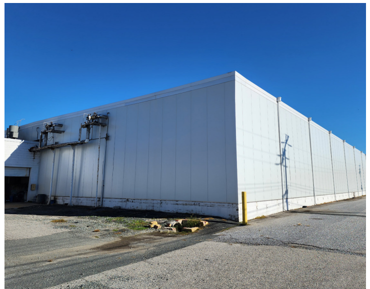
Building 4 ± 12,136 sqft 2 Docks - 26' Ceiling Height
