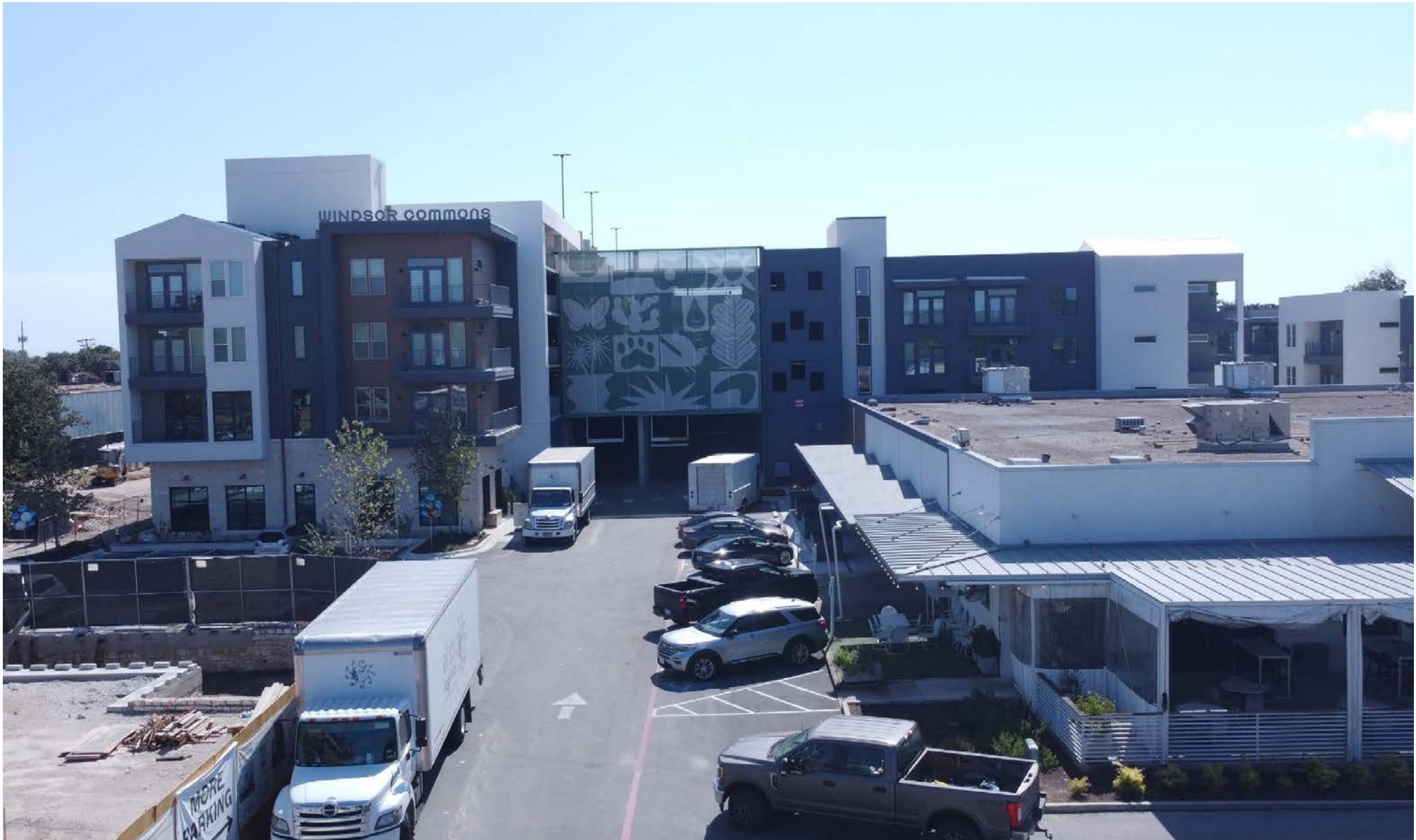
Construction Progression Sep 2024
