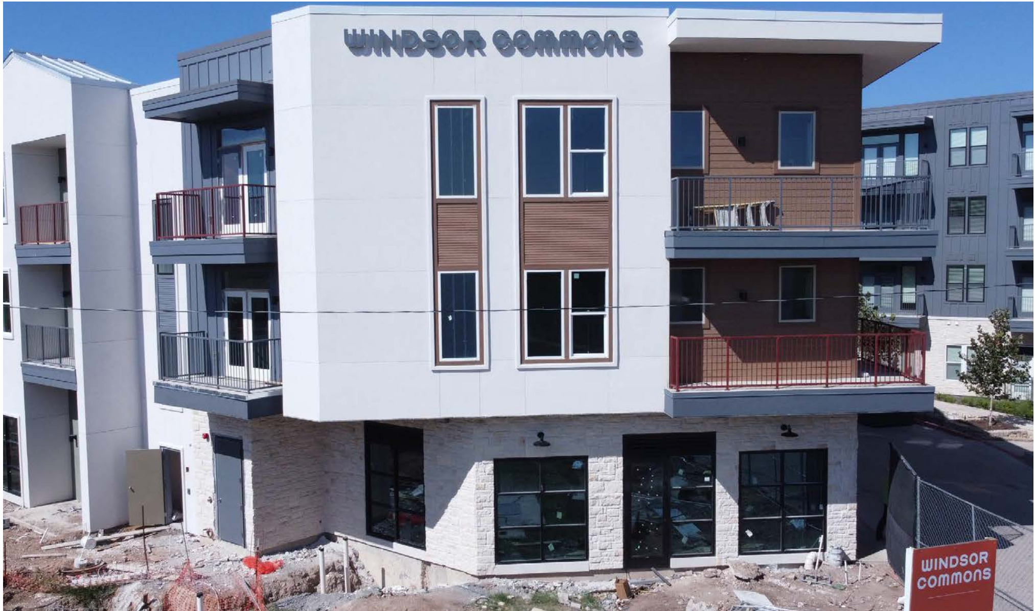
Construction Progression Sep 2024
