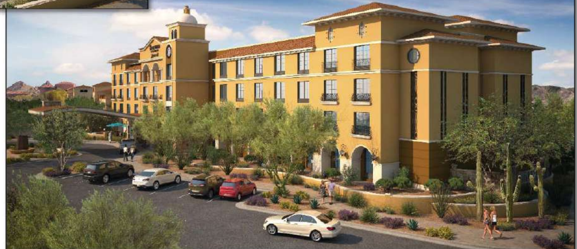
View looking Northeast
