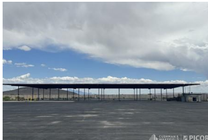
Paved Yard Area
