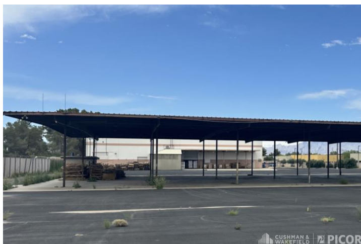
Canopy Area (note—has truck well loading)
