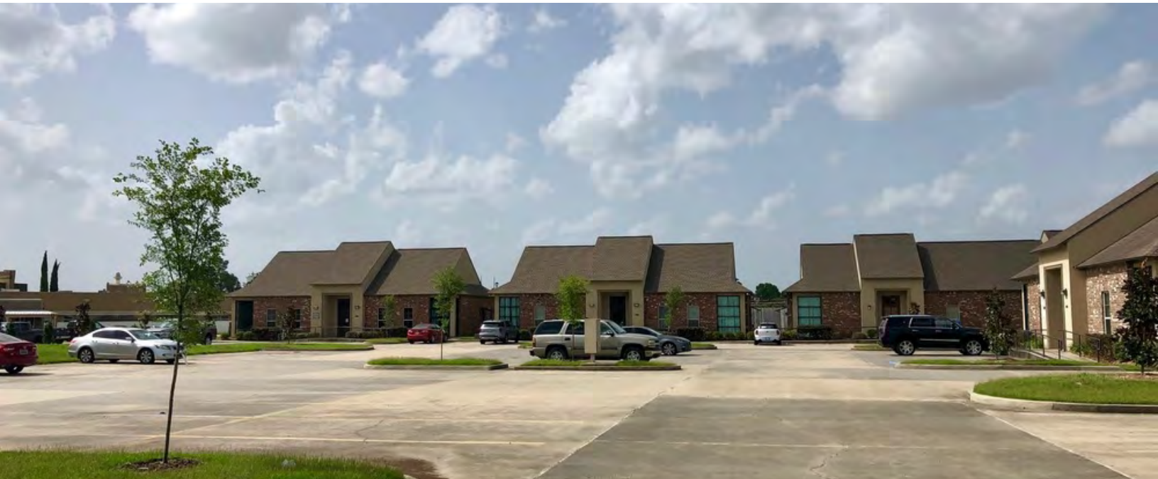
Market Plaza Office Park
