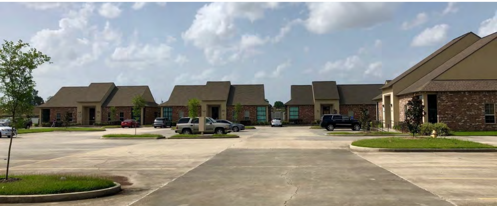
Market Plaza Office Park
