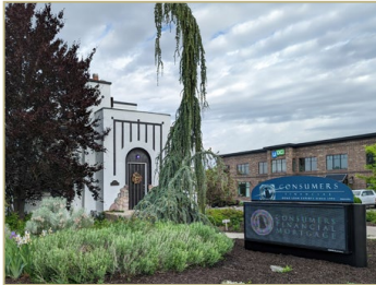
Art Deco Entrance & Monument Sign
