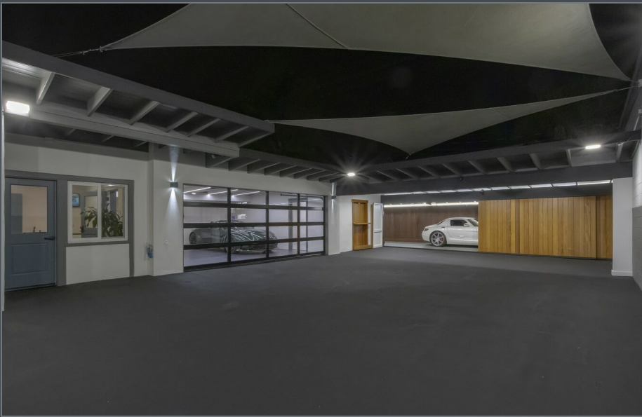
DISPLAY COURT — VAULT DOORS
