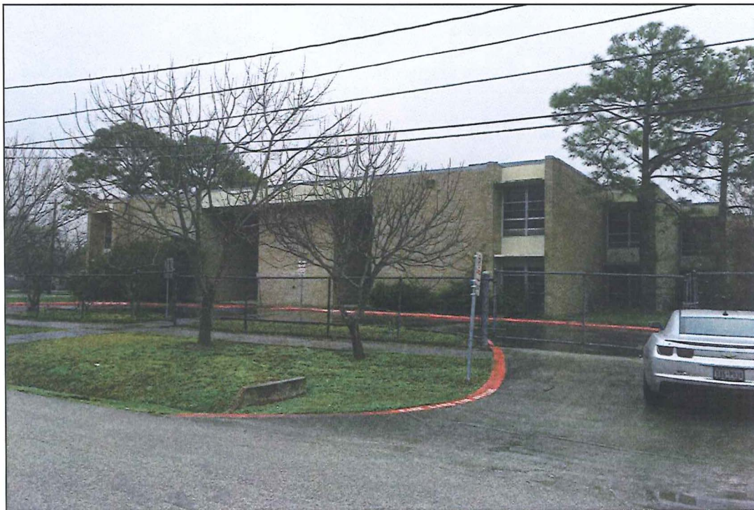
Exterior view of the building looking northeast across Dixie Drive
