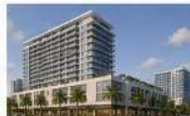
SOLESTE LA PIAZZA YOUNG CIRCLE 23-STORY LUXURY APARTMENTS 378 UNITS UNDER CONSTRUCTION
