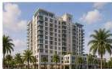
THE TROPIC DOWNTOWN HOLLYWOOD 18-STORY RESIDENTIAL TOWER 223 APARTMENTS UNDER CONSTRUCTION
