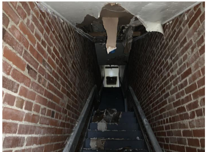
Entrance to Upper Level Apartments
