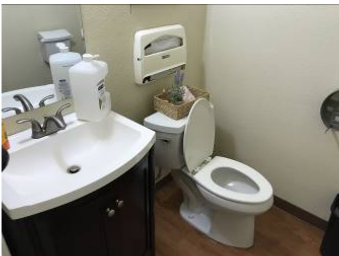
TYPICAL BATHROOM IN 4778 DEWEY DRIVE
