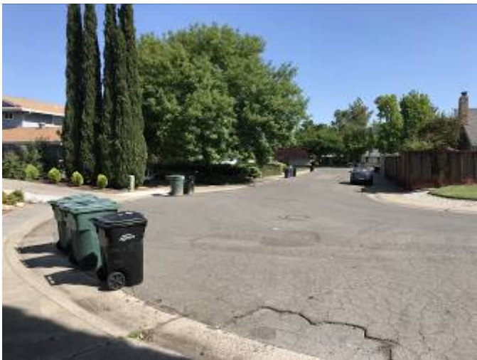
FACING NORTH ALONG SELKIRK WAY
