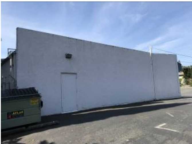
TYPICAL SIDE VIEW OF THE SUBJECT
