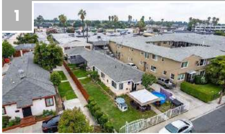
1 3557 BEECHWOOD AVE Lynwood, CA 90262
