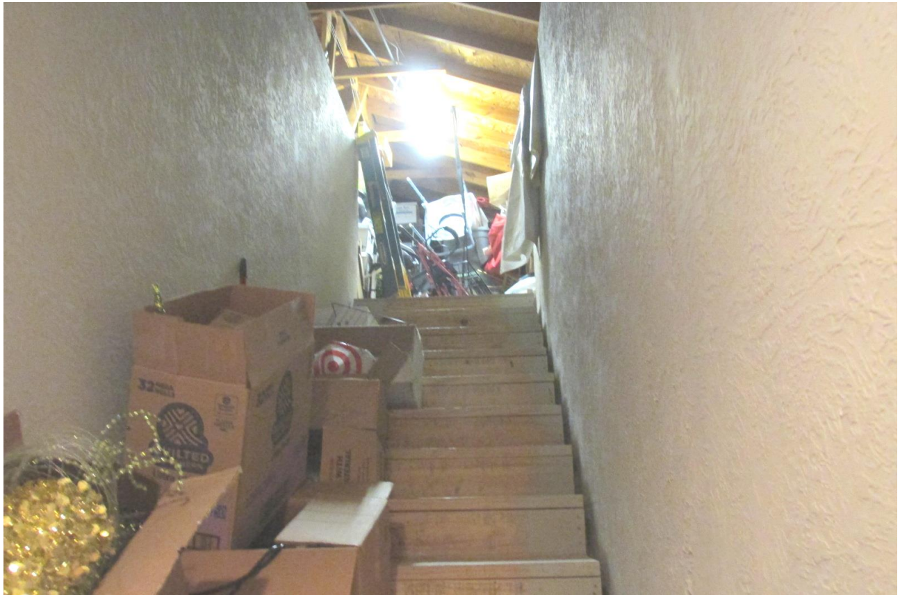
STAIRWAY ACCESS TO FLOORED ATTIC
