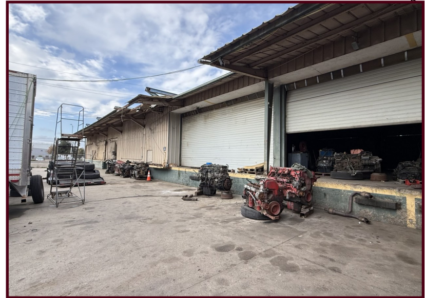
South Side of Warehouse Used by Trucking Company
