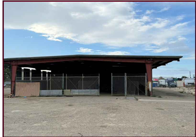
East side of Shop
