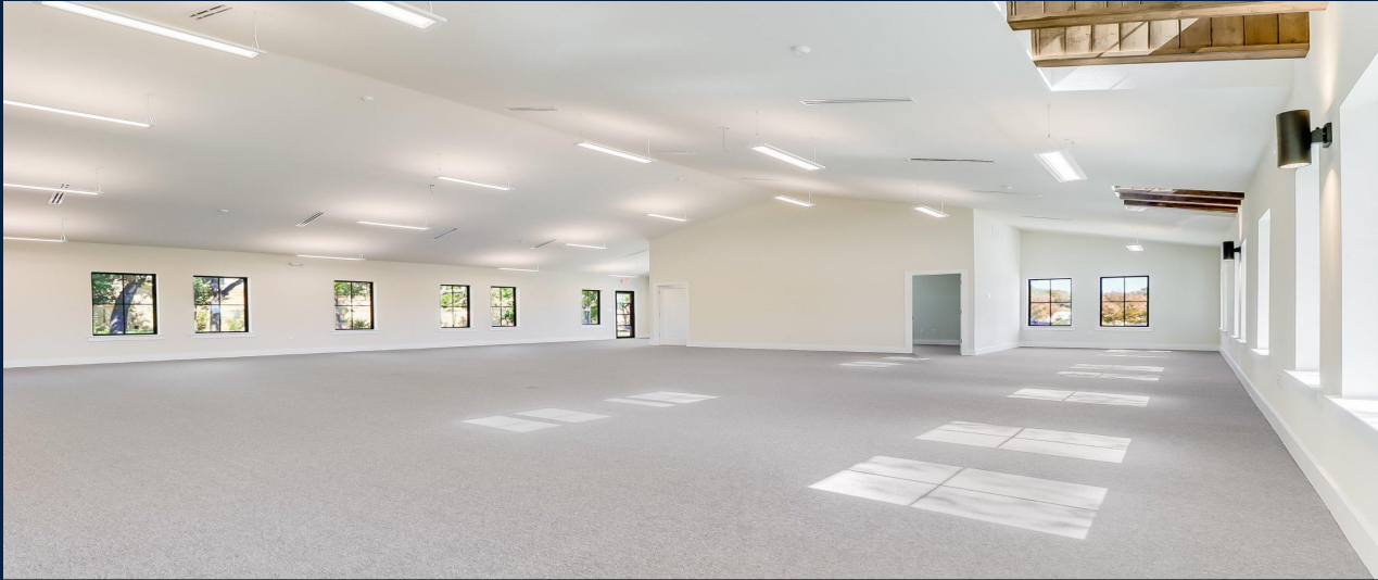
Main Work Area
