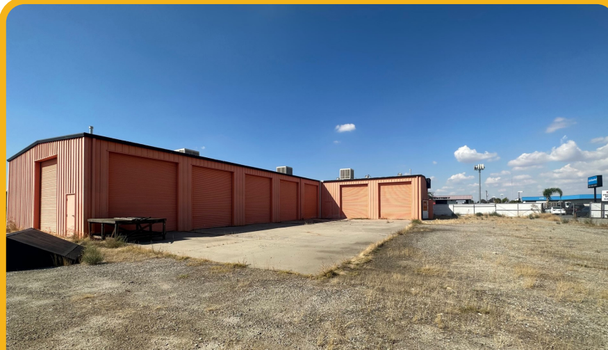
Yard (Concrete & Crushed Rock)
