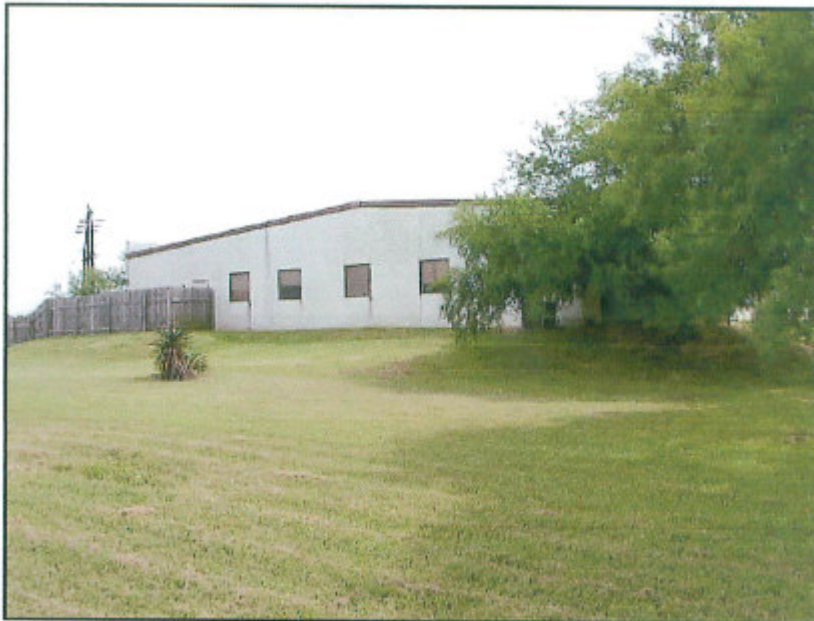
REAR VIEW OF SUBJECT
