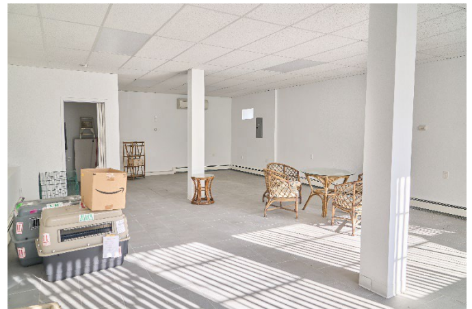
New: Floor & HVAC Split system in ground floor office/retail space
