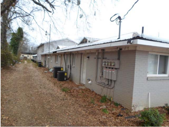
Building 1 - 914 & 916 (Rear View)
