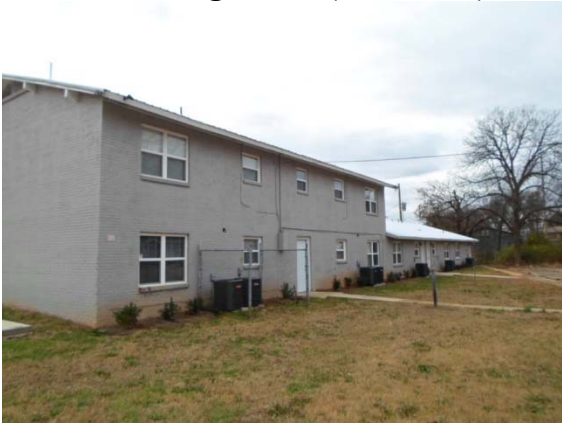
Building 2 - 920 (Rear View)
