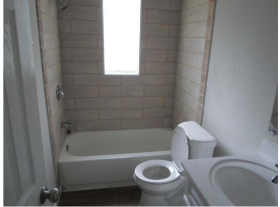
Building 1 - 914-C Interior
