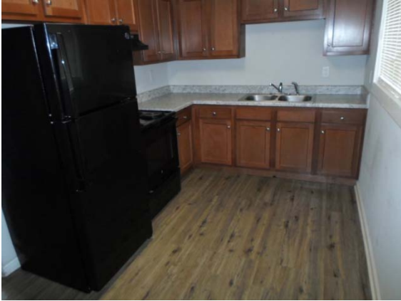
Building 1 - 914-C Interior
