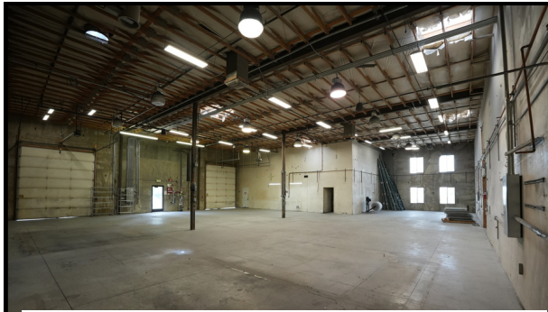
4 flex units - 18' ceiling height
