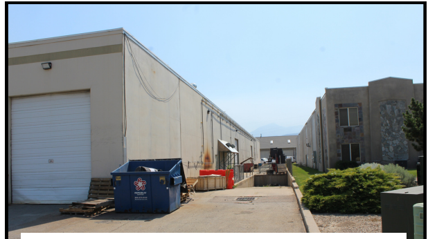
Shared loading dock
