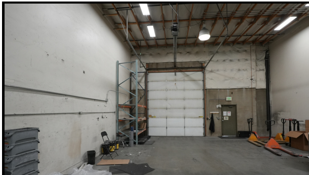
7 ground level doors (12'x14')
