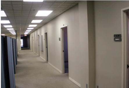
Typical Office Finish
