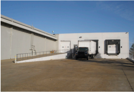
Main Dock Doors and Ramp
