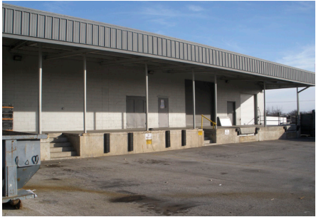
West Side Truck Court
