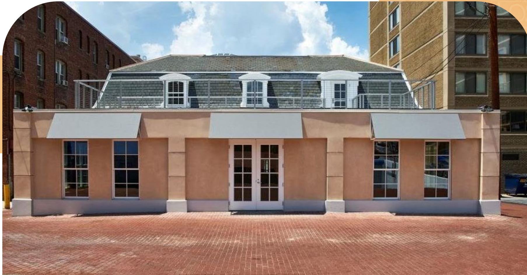
BACK OF BUILDING
