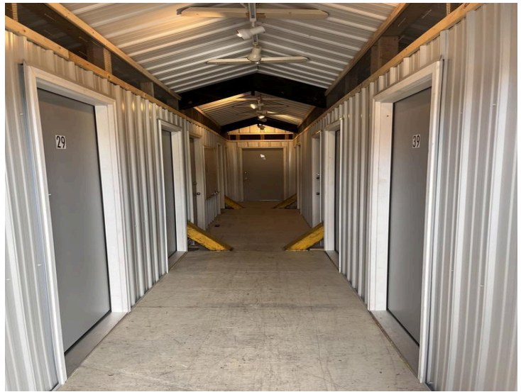
Upper-Floor Storage / Apartment Wing Hallway
