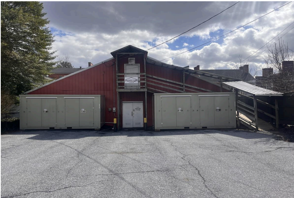
Self-Storage Facility — Exterior (150 W Market St)
