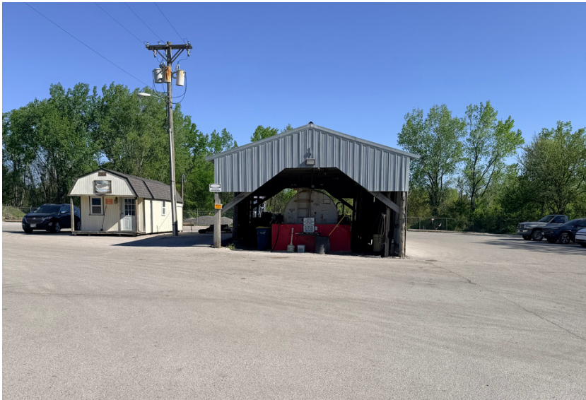
Covered outdoor storage
