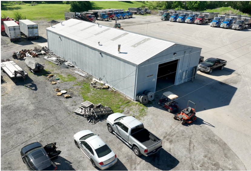
3,600 SF building with drive-thru capability
