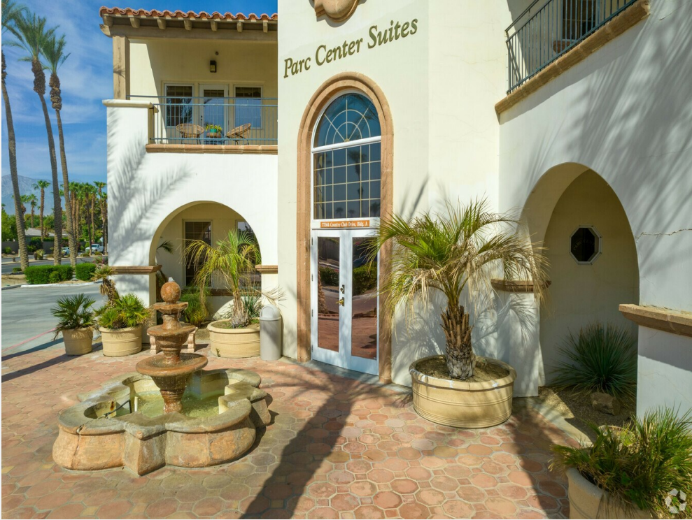
This Office/Showroom Facility Holds Lush Landscaping, Peaceful Mountain Views, in a Desert Oasis
