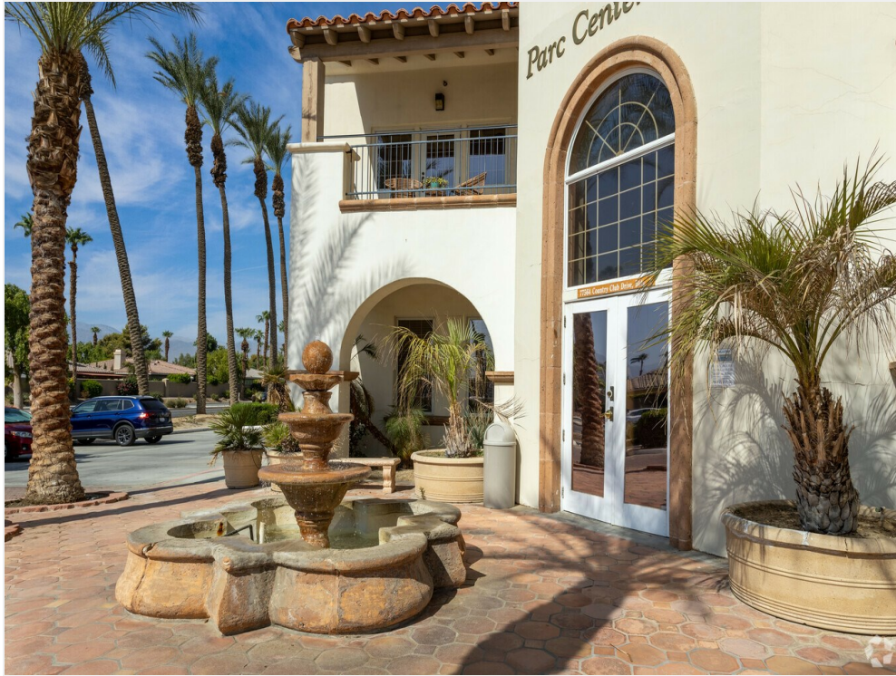
This Office/Showroom Facility Holds Lush Landscaping, Peaceful Mountain Views, in a Desert Oasis
