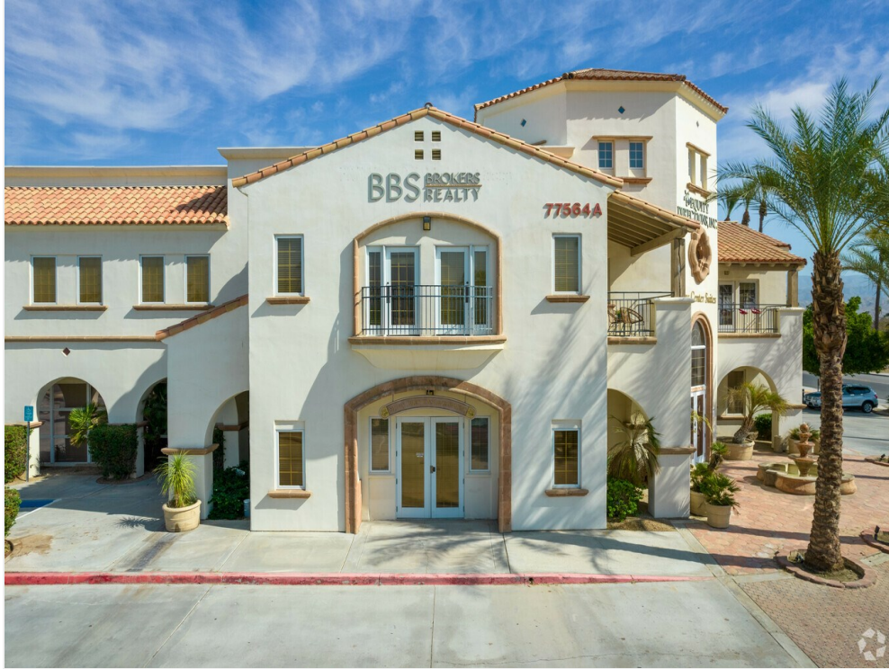
Park Center Business Park a Professional Environment with California Mission and Traditional Mediterranean Architecture
