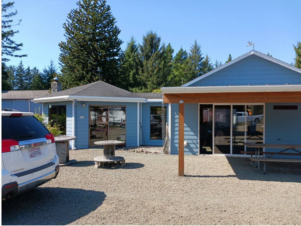
Enclosed Gazebo, with a wood stove, and Dining Area
