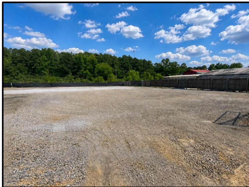
Ground surface is mostly flat with packed gravel
