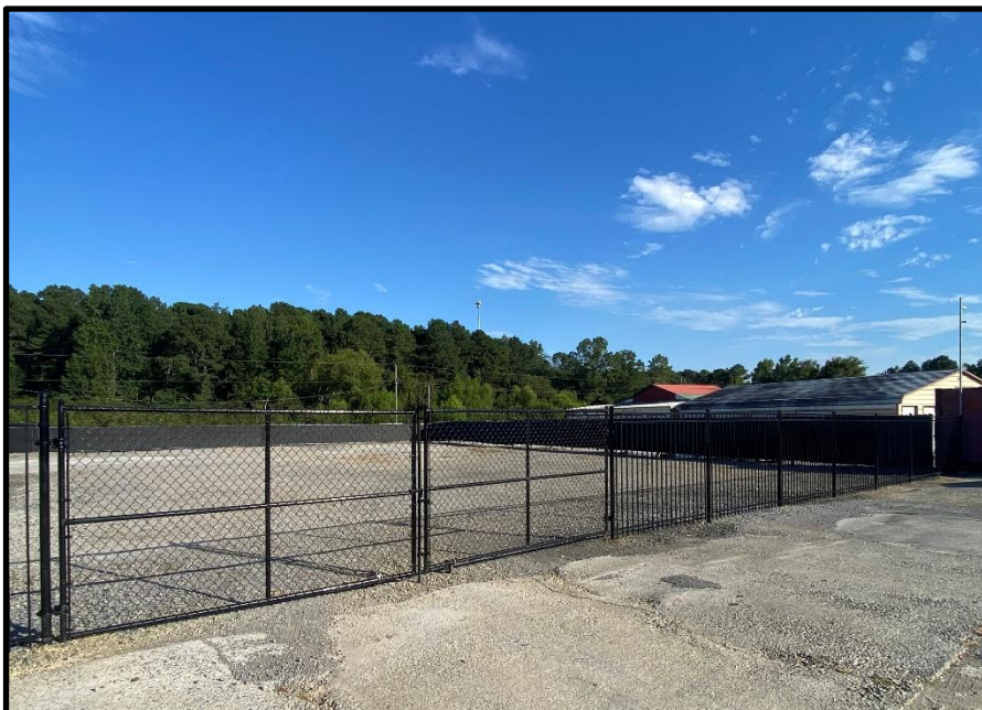
Perimeter fencing with 24ft wide lockable metal gates
