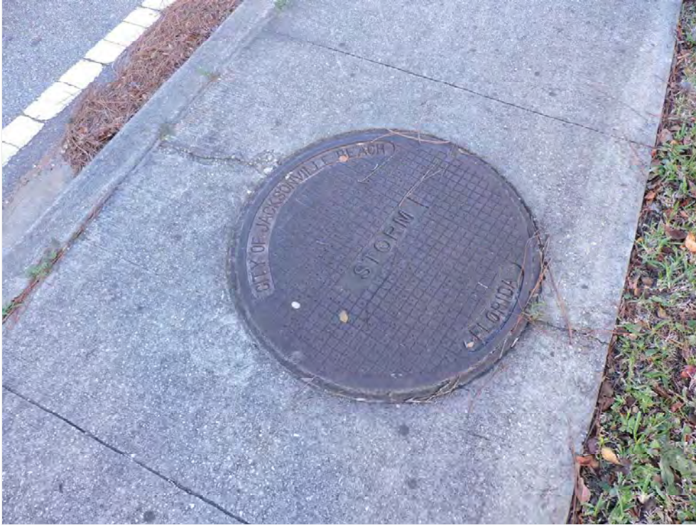
Storm Sewer at Yellow Bluff
