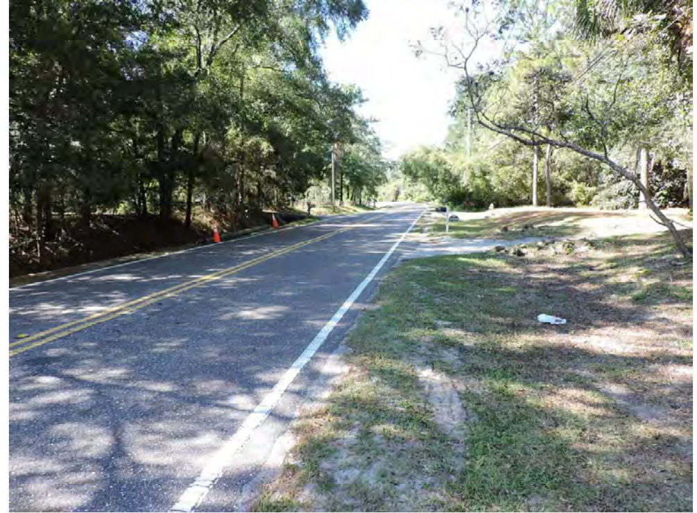
2955 New Berlin (13) Road Frontage to West
