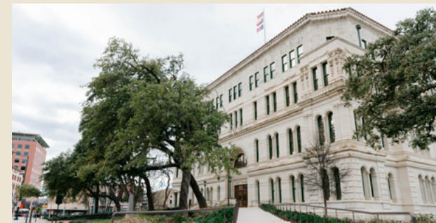
CITY HALL As one of the nation's oldest public buildings, San Antonio City Hall is been home to more than a century of civic action.
