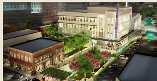
ALAMEDA THEATER The Alameda Theater, next to the San Pedro Creek, has been undergoing restoration. It is slated to re-open to the public in 2026.
