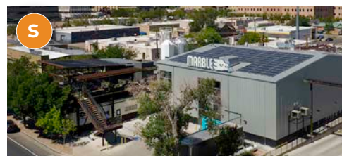
111 Marble Ave NW 102 Granite Ave NW | 1021 1st St NW
