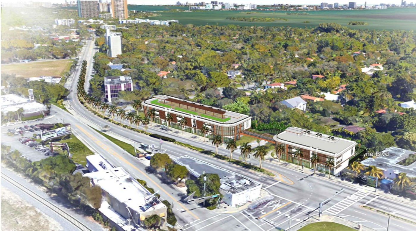
Southwest Aerial | North Building (5501) and South Building (5445)
