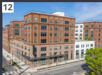
12 LC SOBRO Apartments + Retail Completed May 2020
